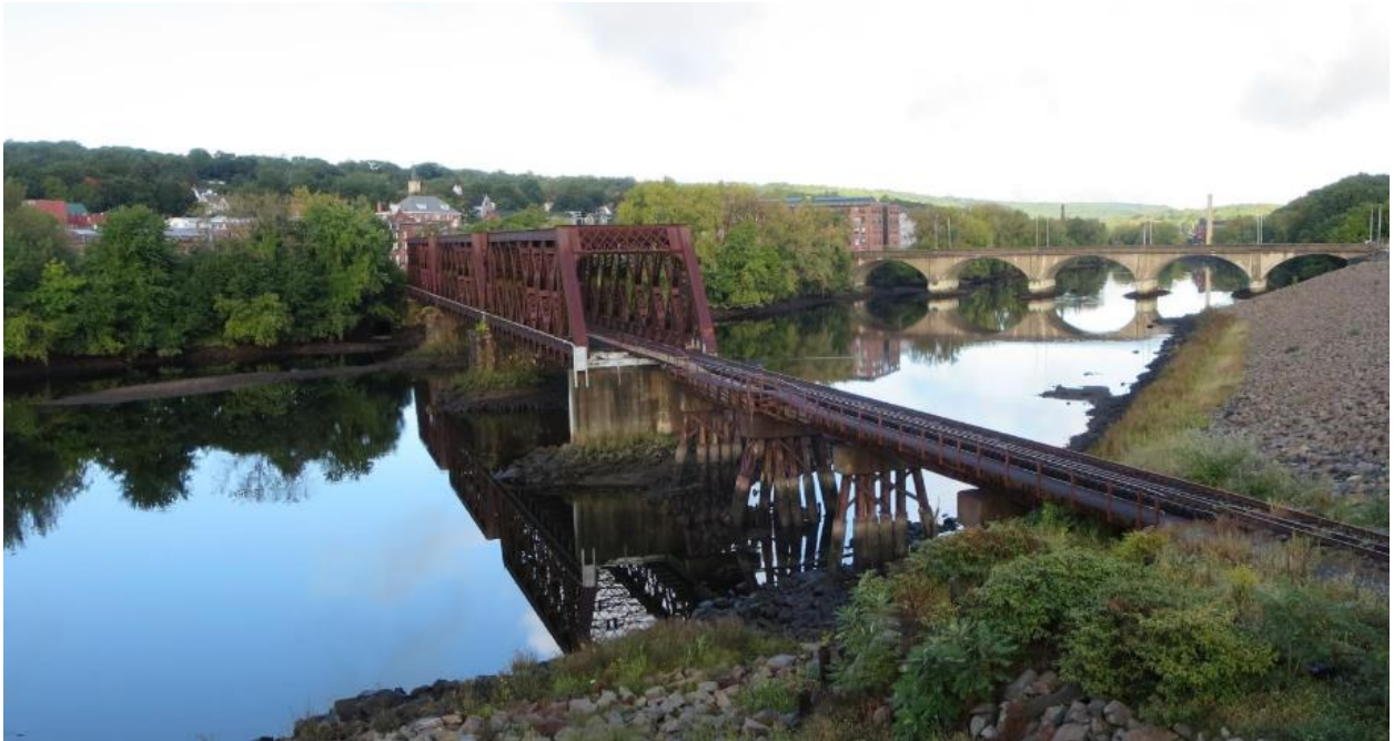
Figure 4.8 Historical Rail Bridge in Derby, CT
