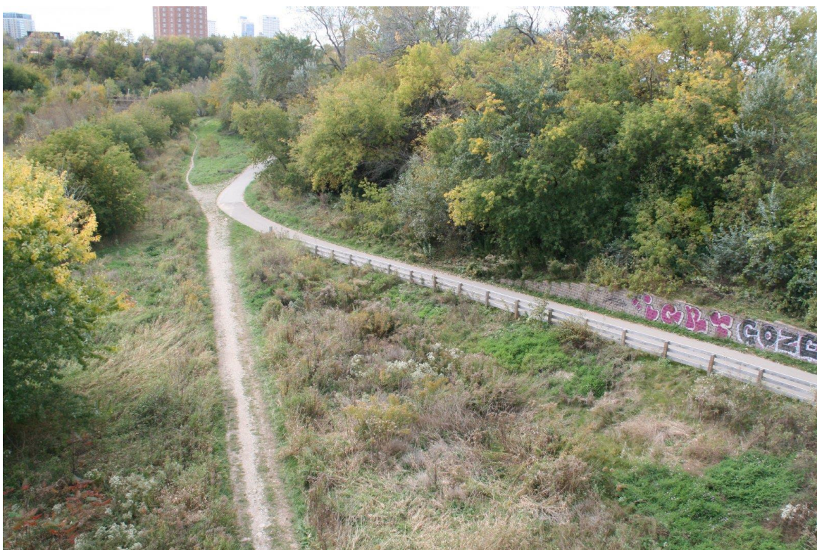
Figure 4.16 Beerline Trail alongside old rail line
